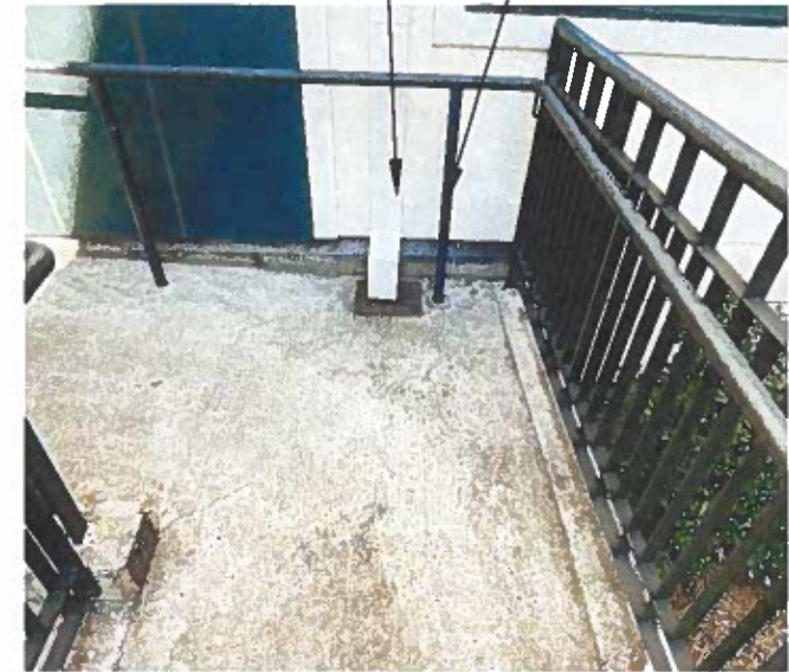
EXISTING RAMP & HANDRAIL SCALE: N.T.S. (AT COURTYARD)
